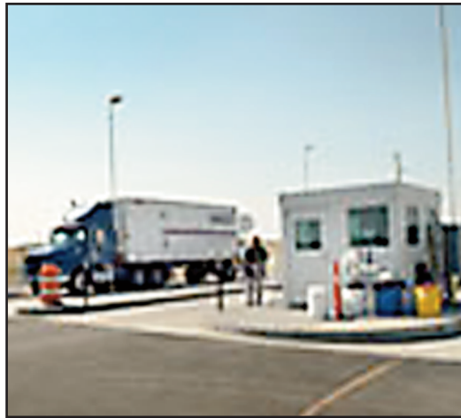
Security checkpoint at Columbia Generating Station.
